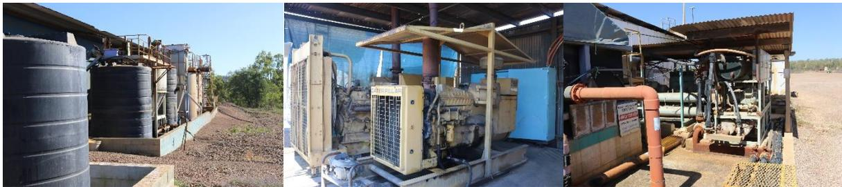
*Figure 1. (a) Civil works will include repair of the existing bunds (b) side by side generators and (c) Generator and chiller compressor housing.*
