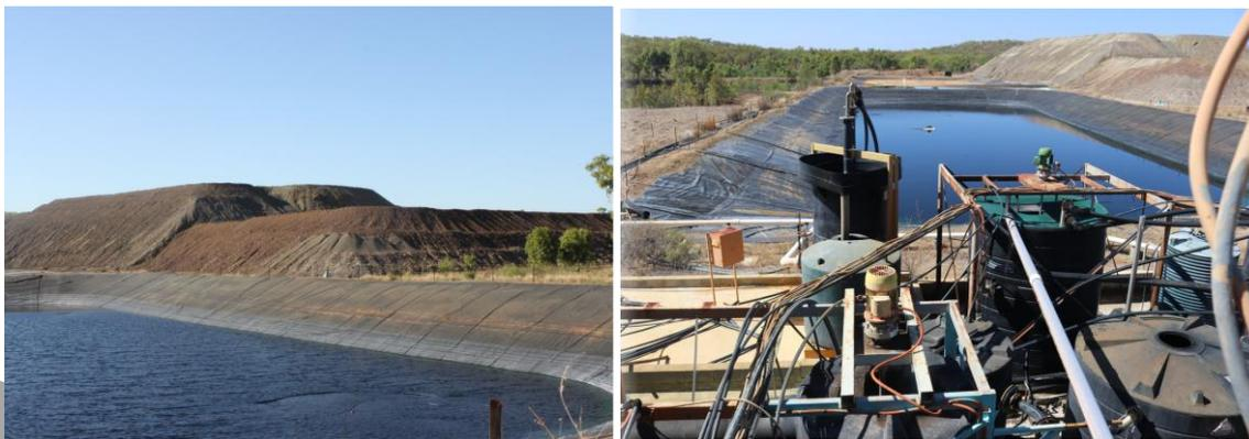
Figure 2. Heap leach pads and part of the plant with ponds in the background.
